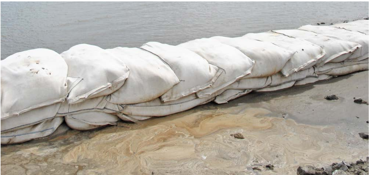
Figure 4: Temporary flood protection structure made of 1 m 3 sand containers
