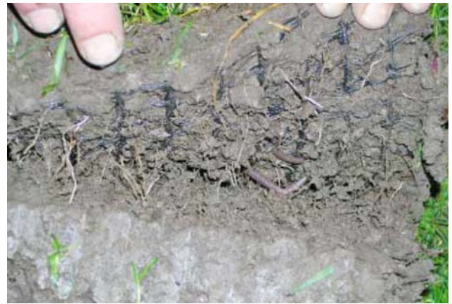
Erosion control grid with ingrown turf, taken from [14]
