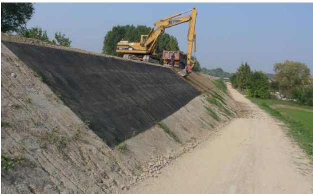
Figure 12: Erosion protection grid during installation;
