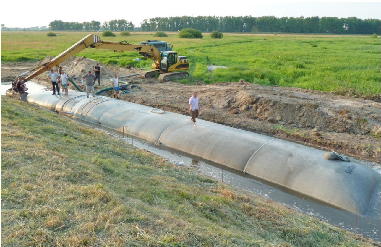
Figure 5: Geotextile tube during filling
