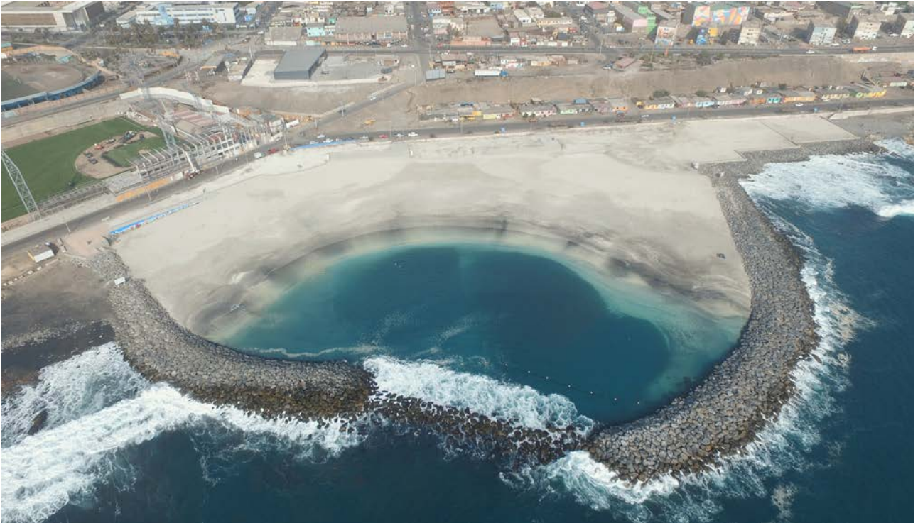
Picture 7: Beach in Tocopilla after completion
