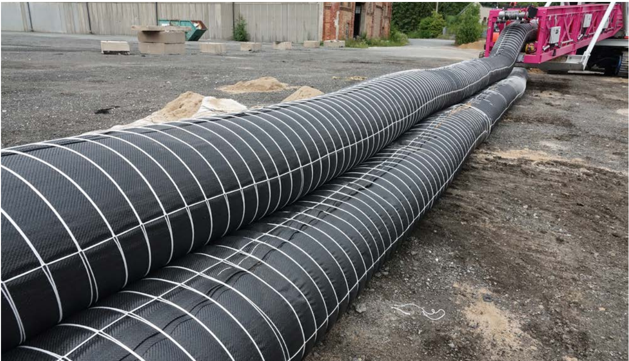
Figure 9: Tube from a tube paver
