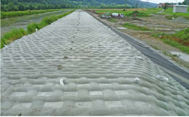
Figure 13: Concrete mattress after installation;
