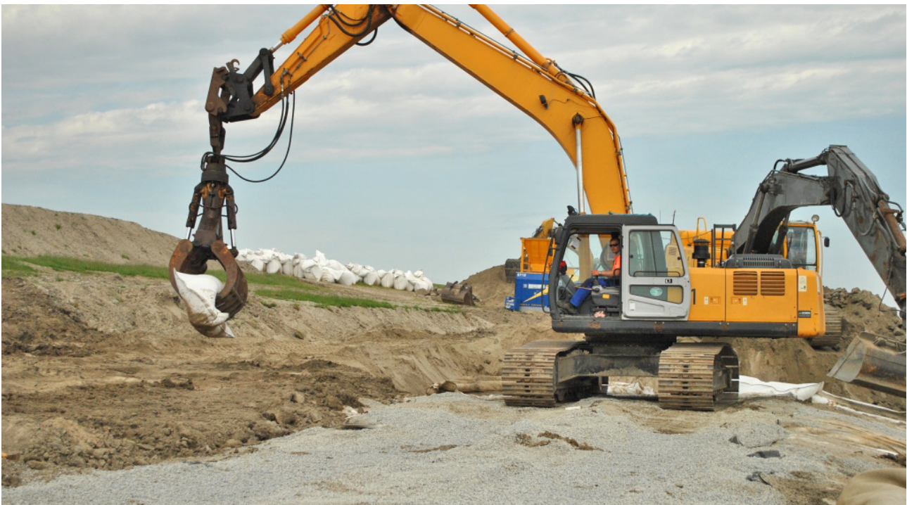
Figure 3: Transportation and laying of large sand containers
