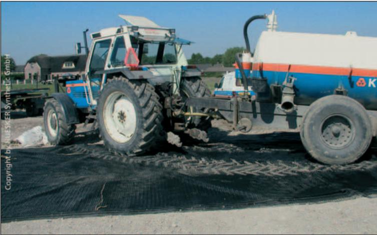
Figure 9. Improper storage / treatment of unrolled geogrids
