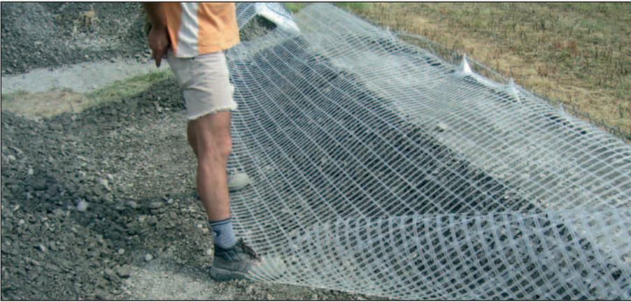
Fig. 11. Memory-effect of interlaced geogrid
