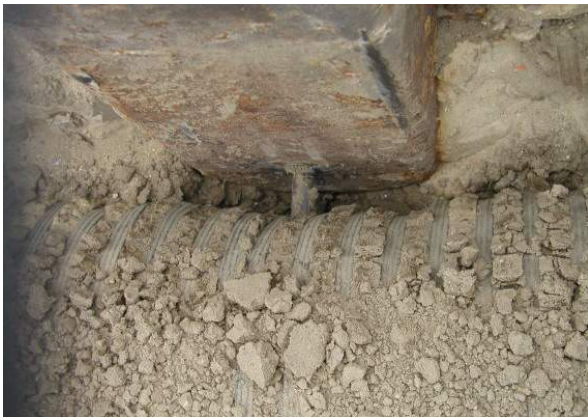
Fig. 6 Connection detail and the tensioned geogrid
