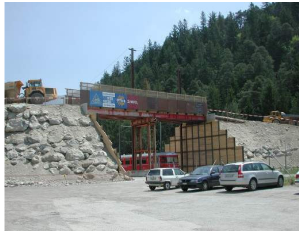
Fig. 1 Temporary bridge with geogrids as anchor elements
