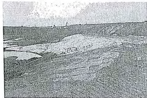
Figure 4. Profiling the slopes to 1v:3h.
