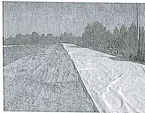
Figure 14. Preparation of the panel on site.
