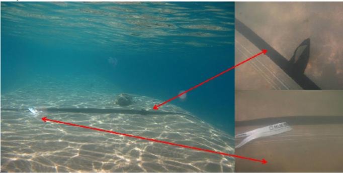
Figure 7 Marks on tube surface
