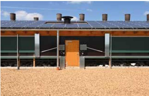
Lubratec bottom-opening wrap-around ventilation with electric drive
