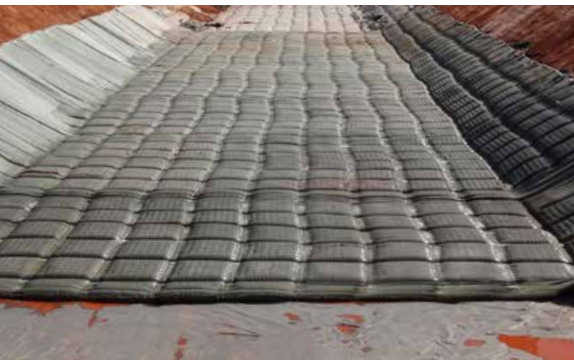
Canal construction Brazil | Lining of a canal bed using Incomat Flex.
