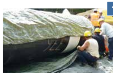
Fixing to pipe section
