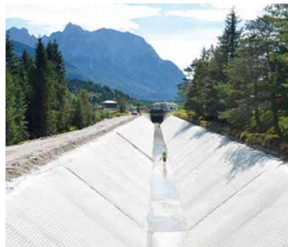
Canal renovation Germany | Lining of the Isar link canal using Incomat Standard geosynthetic concrete mattress.
