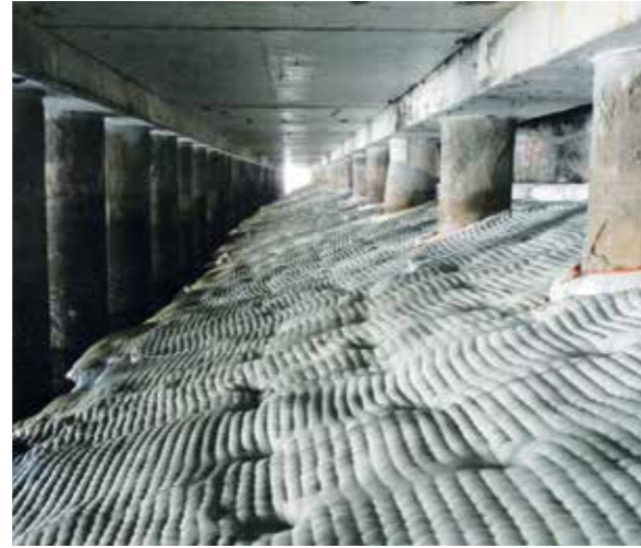
Berth protection Guatemala | slope and berth protection at the new port terminal of Puerto Quetzal using Incomat Standard.
