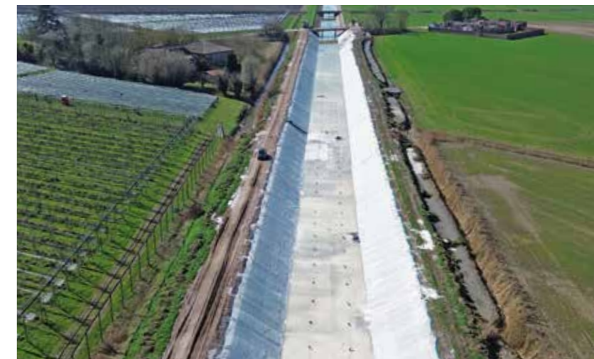
Channel lining Italy | Sealing an irrigation channel using Incomat Standard.
