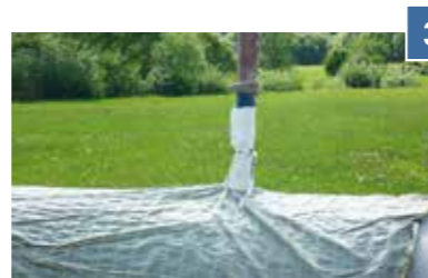
Concreting via filler neck
