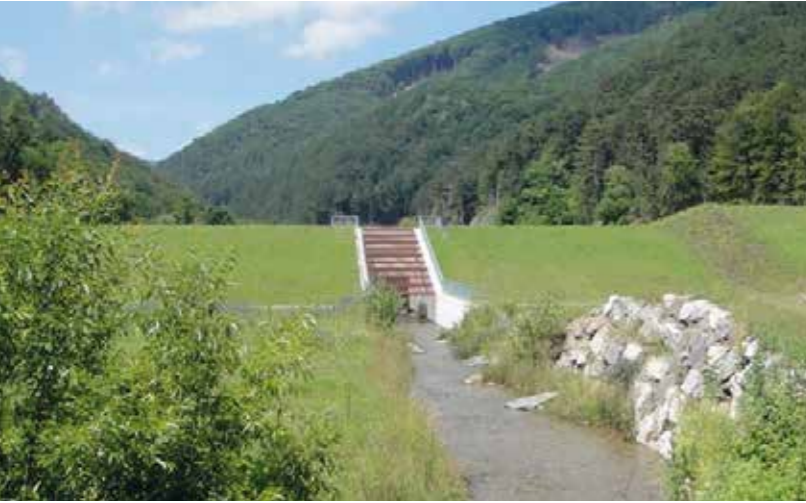
Overflow section Austria | Erosion protection in an overflow section using Incomat Crib.
