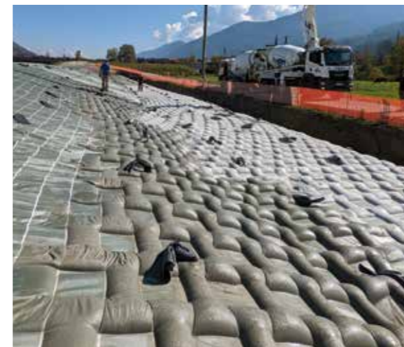
Erosion protection Austria | Erosion protection of a overtopping spillway using Incomat Crib.
