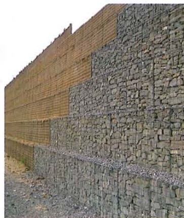
Unfilled row of gabions tied back with geogrids from Huesker
