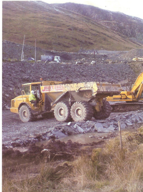
Ground improvement along the A470 using slate fill
