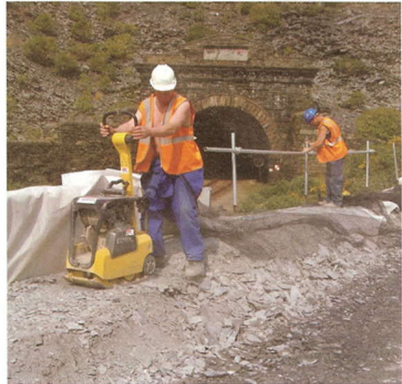
Slate fill is compacted in layers up to 600mm deep along the temporary diversion
