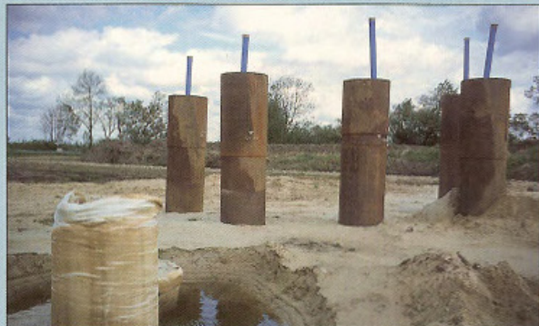
GEC columns are being trialled for a showpiece bridge.
