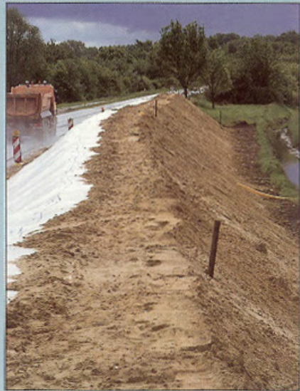
Vast amounts of sand surcharge accelerate settlement on the route.
