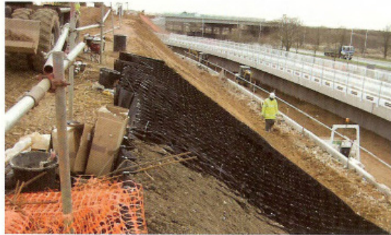
The complex slope profiles vary from 26° to 64° as the embankments near the tunnel under the roundabout.
