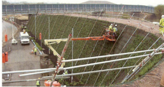
The complex slope profiles vary from 26° to 64° as the embankments near the tunnel under the roundabout.
