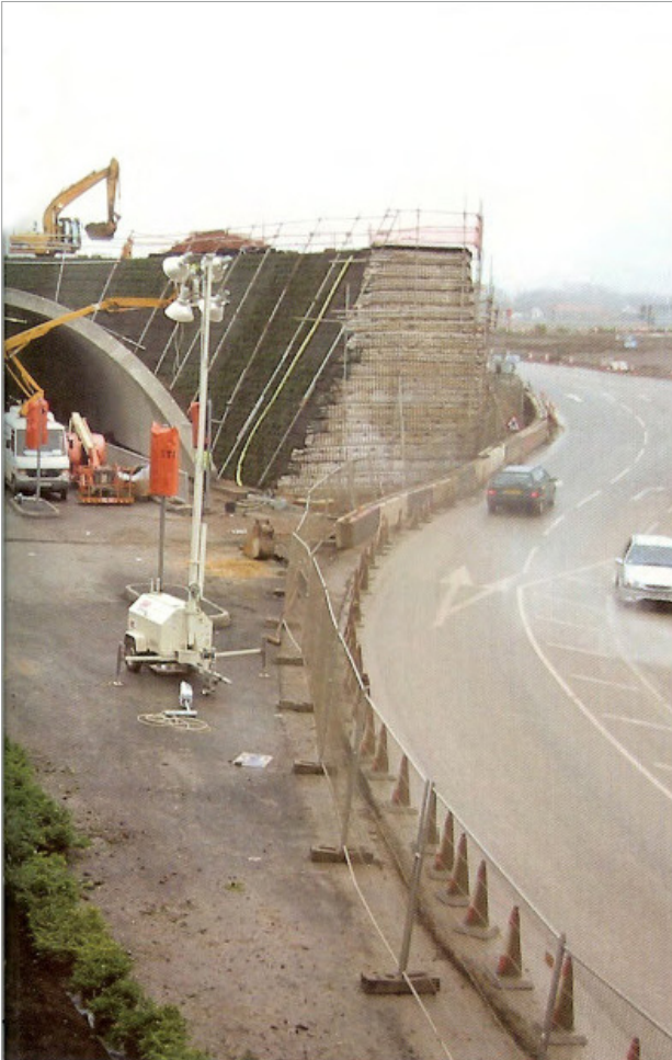
The complex slope profiles vary from 26° to 64° as the embankments near the tunnel under the roundabout.
