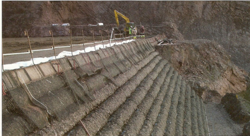
Pascoe modified the layout of the embankment to work better with the rock contours
