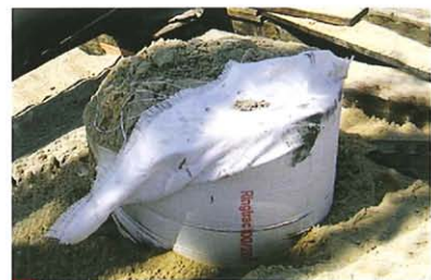
Figure 6 Recently installed sand-filled geotextile-encased column (GEC) using Ringtrac® 100/250.
