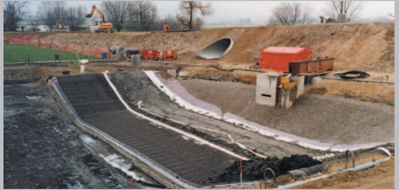
Settling lagoons - Lining with NaBento®
