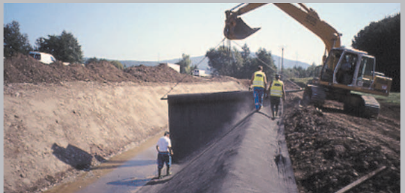
River-bed lining with NaBento®
