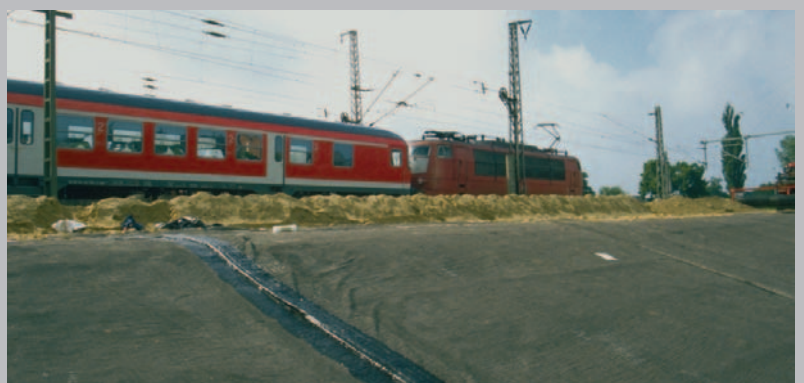
Railway lining with NaBento®
