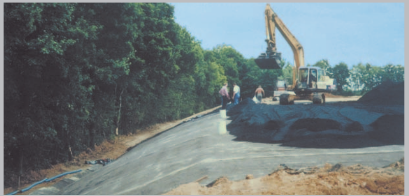
Landfill capping with NaBento®
