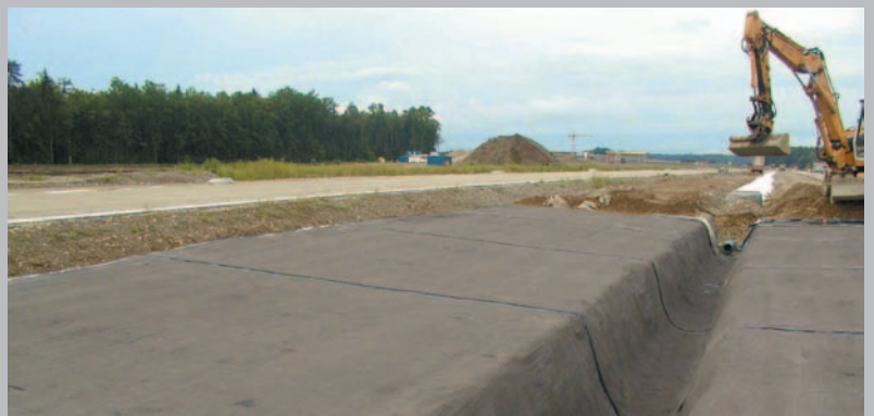
Groundwater protection on a road scheme
