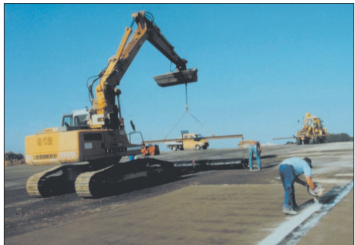
NaBento®- installation in a landfill construction
