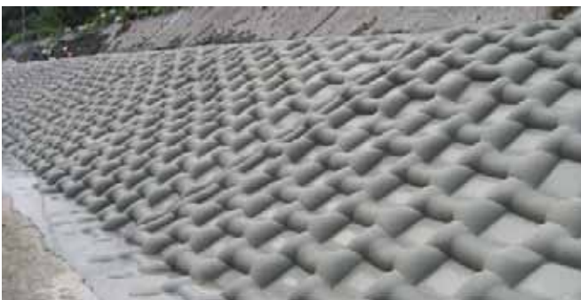
Incomat® Crib a tubular grid profile mat with unfilled central apertures for technical/environmental slope protection above the permanent water surface, especially where establishment of vegetation is desired.
