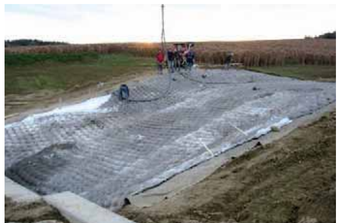
Incomat® FP after filling with concrete (2)
