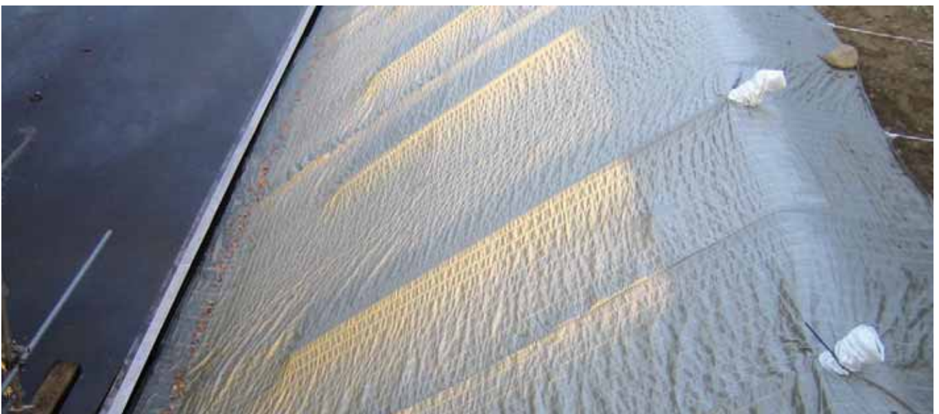
Incomat® Standard panels prepared for filling with concrete.
