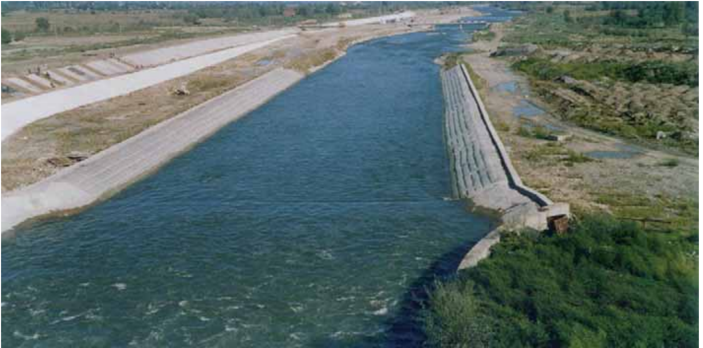
Slope protection with Incomat® Flex
