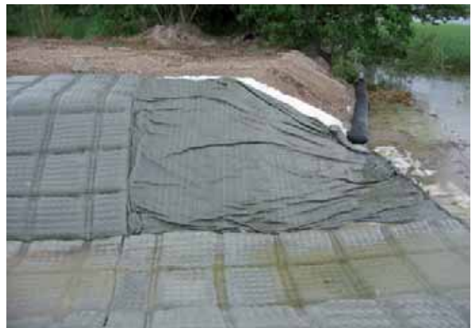
Installation (filled and unfilled section) (3)
