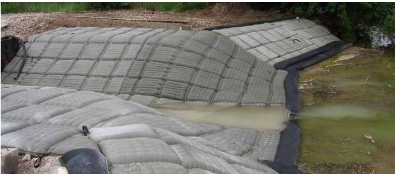
Repaired outlet after completion (4)
