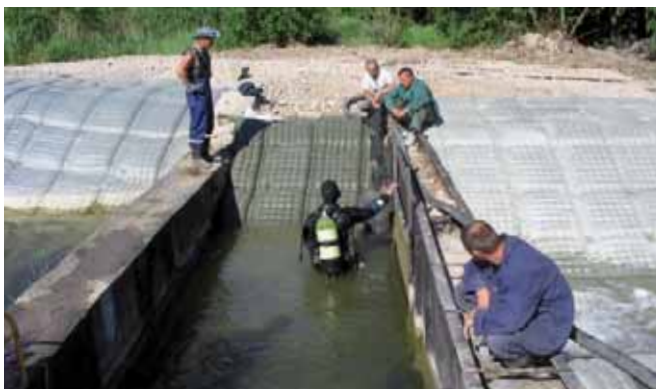
Installation of Incomat® Flex under water
