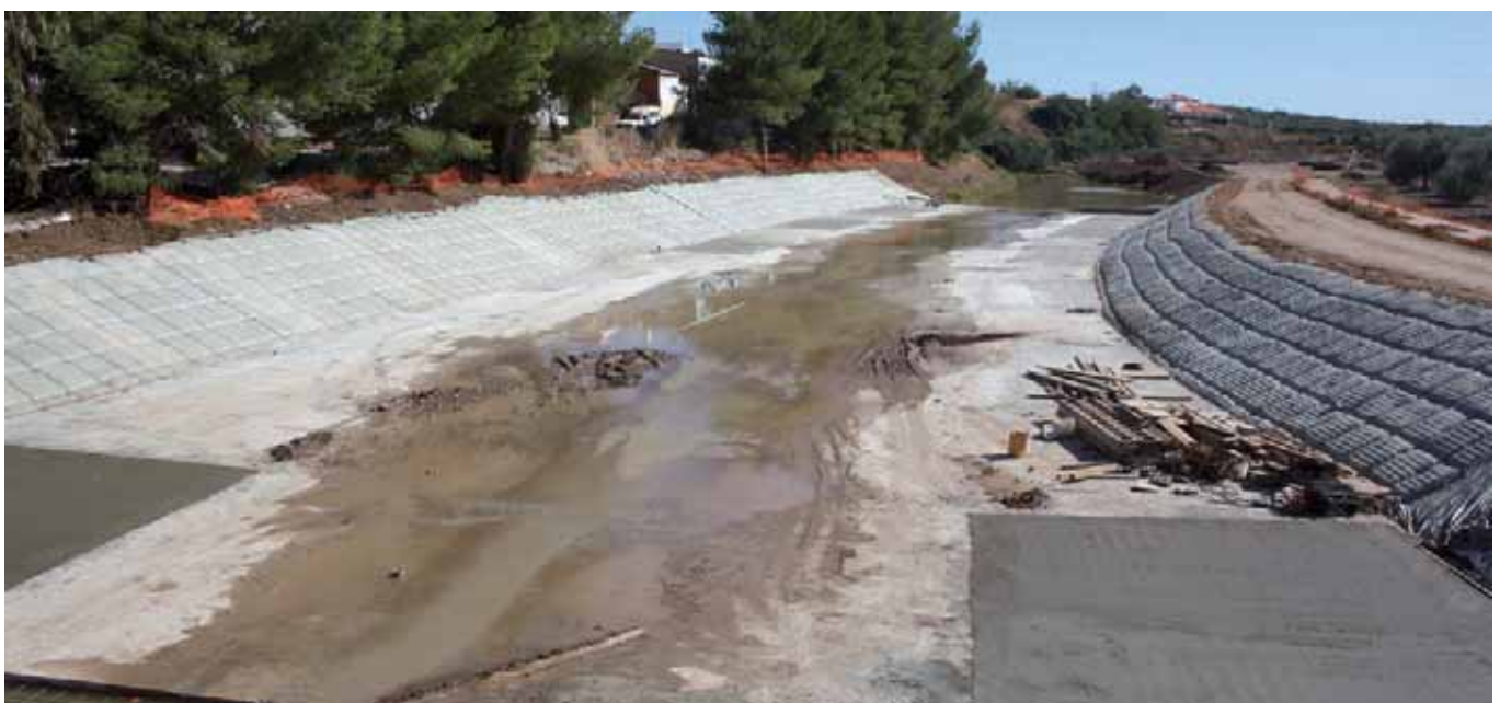
Slope protection with Incomat® Flex
