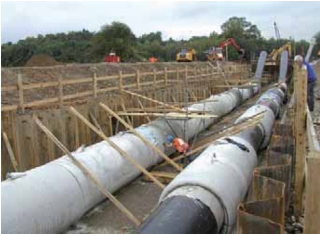
Incomat® Standard as a negative buoyancy collar for an inverted siphon system
