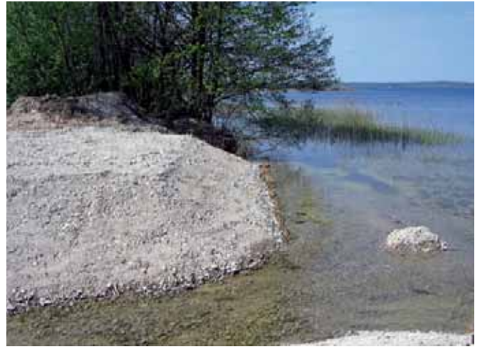
Slope preparation (earth works) (2)
