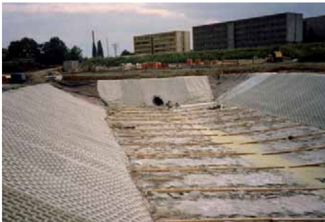
Attenuation pond with Incomat® Crib during construction (1)
