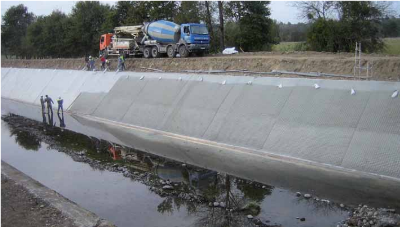
Progressive filling process of Incomat®
