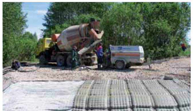
Installation of Incomat® Flex
