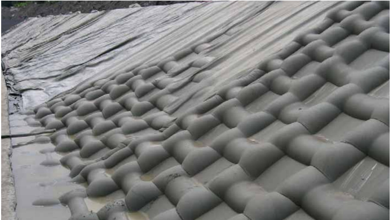
Installation of Incomat® Crib
