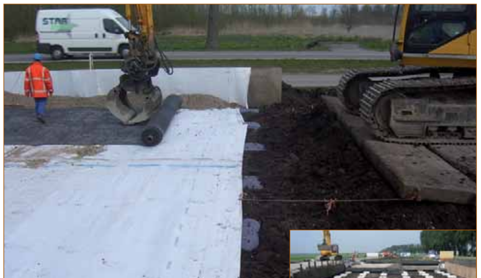
Piled embankment, Project: N210, NL
