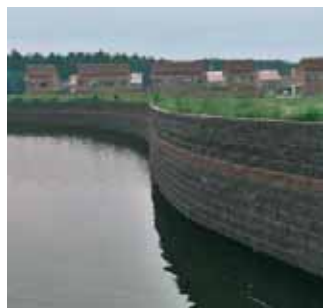
Segmental Retaining walls
