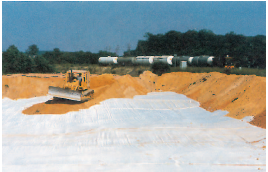
Once installed, the fabric was strong enough to give support to 4 t bulldozer laying fingers of fill material during the initial fill process.
