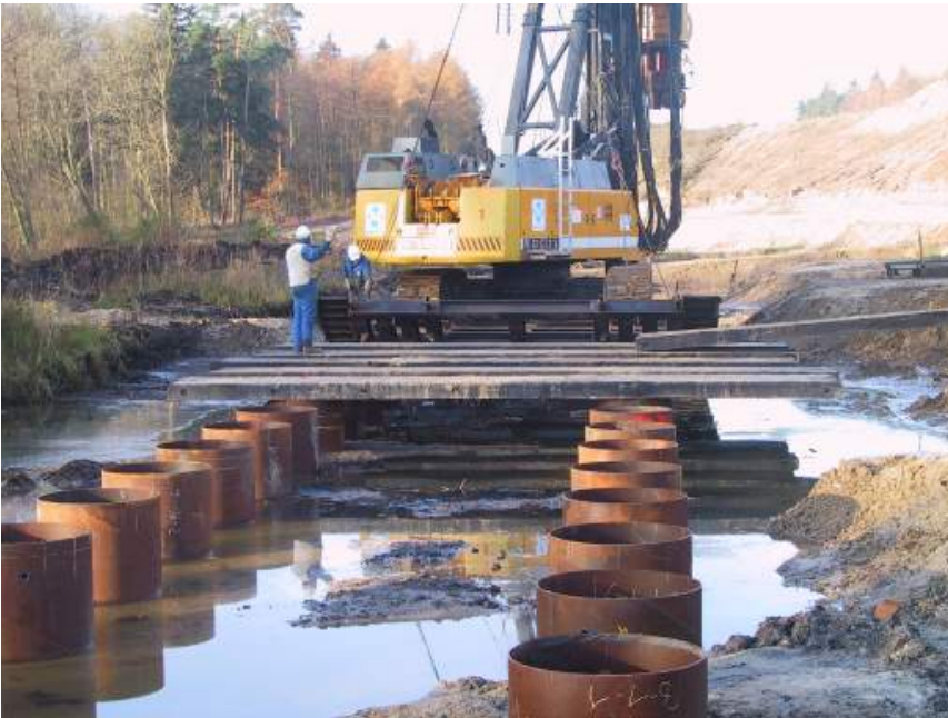
Figure 7. Installation plant on the installed steel tubes (photo: Möbius)
