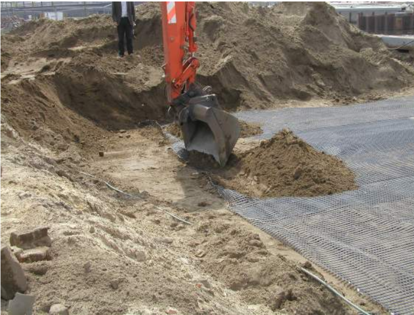
Figure 3. Tensioning the geogrid with the shovel of an excavator (photo: Huesker)
