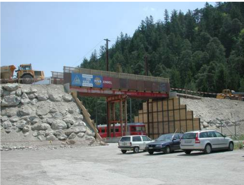
Figure 5. Finalised bridge under traffic (photo: Schoellkopf)
